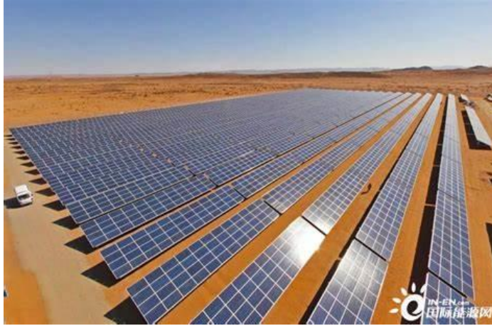
Figure II.12 : centrale solaire photovoltaïque [61].
