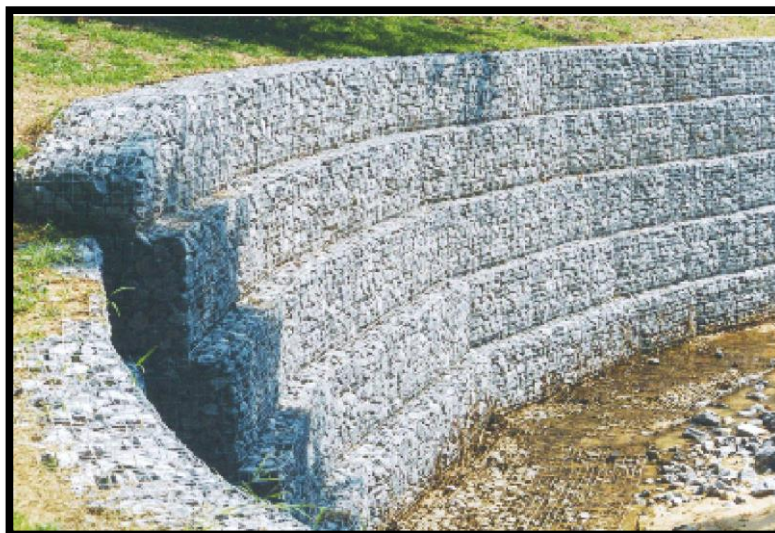
Figure 3.26: Gabion wall. ( http://galleryhip.com/ )
