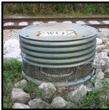
Figure 3.14: relief well. ( http://www.earthcityld.com/floodc.aspx )
