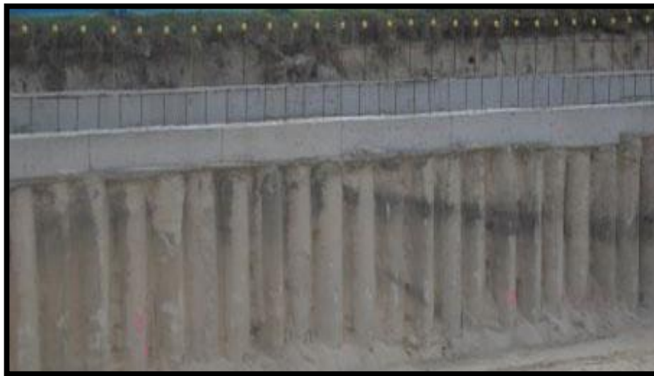
Figure 3.33: Pile Wall. ( http://www.aiclasspiling.com.au/ )
