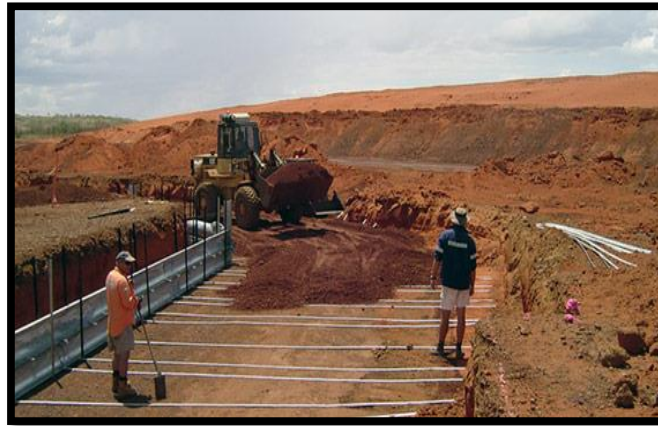
Figure 3.27: Reinforced earth. ( http://www.retainingsolutions.com.au/ )
