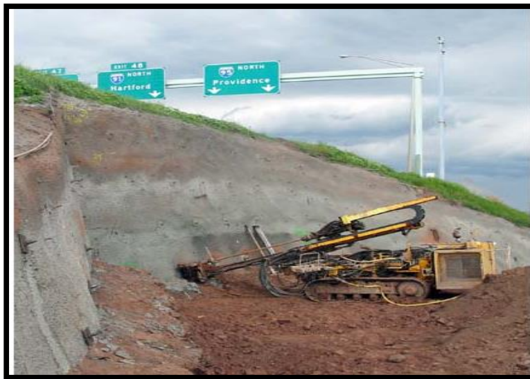
Figure 3.20: Soil nailing and shotcrete. ( http://www.haywardbaker.com )
