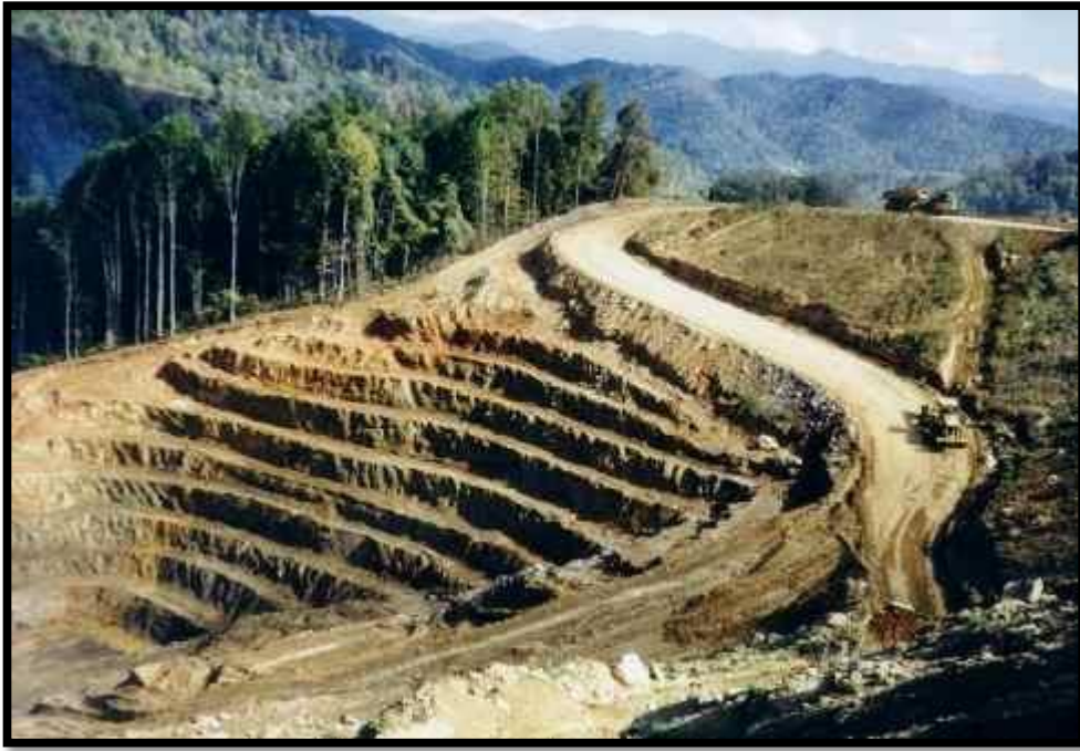
Figure 3.6: benching the slope. ( http://a10.jlansford.com )
