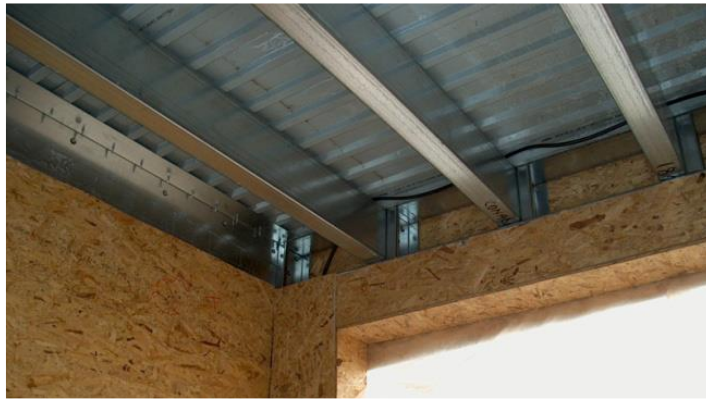
Figure 1.14 : solives de plancher
