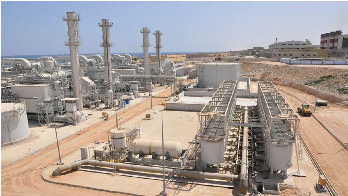
Figure 15 : ZAWIA DESALINATION PLANT IN LIBYA (ENKA, 2025)
