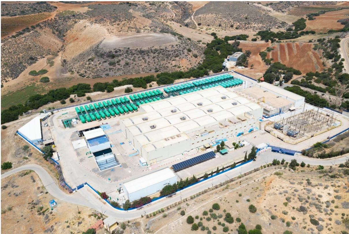
Figure 10 Beni Saf water company: a seawater desalination (BWC, 2025)
