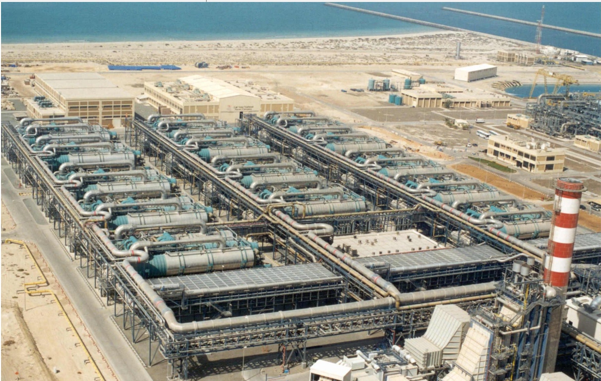
Figure 2: Ras Al-Khair Desalination Plant in Saudi Arabia (UTILITIES, 2025)
