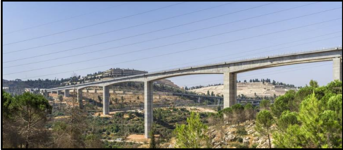
Figure 10: Continuous balanced cantilever bridge
