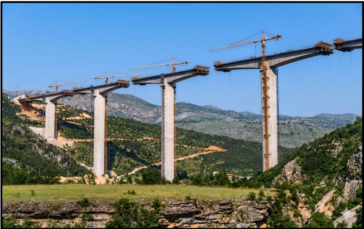
Figure 1: Construction of a long-span prestressed concrete bridge using the balanced cantilever method.
