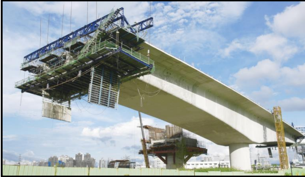
Figure 17: In situ concrete method
