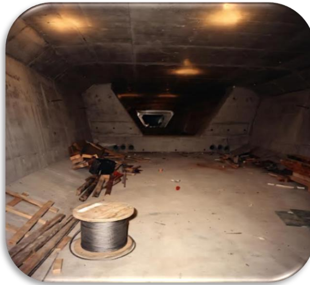
Figure 31: Interior View of a Span deviator Within the Box Girder
