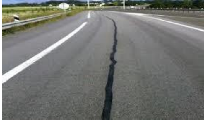
Figure 29: Fissures d'adaptation [5].
