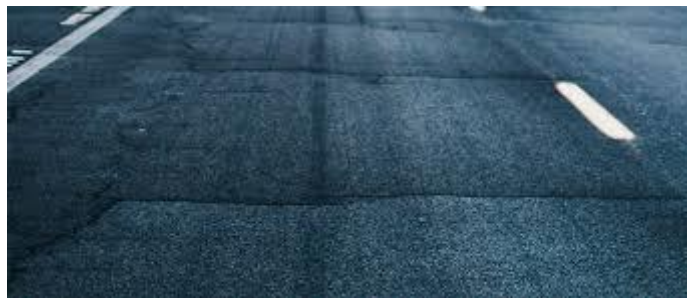
Figure 25: Fissures transversales [5].
