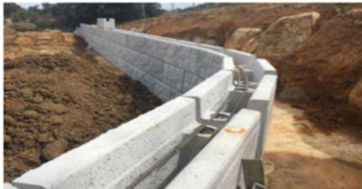
Figure 2.21 : Mur en cantilever (Youcef tani. & ramdani., 2021)
