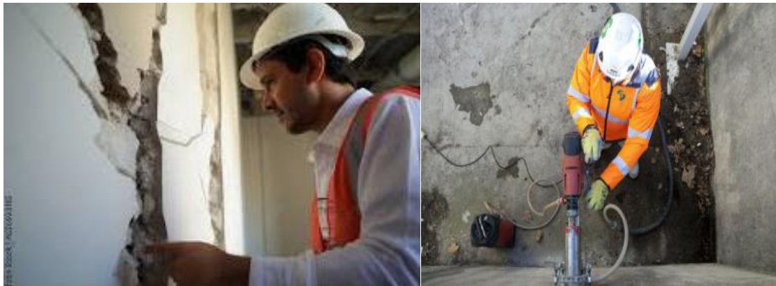
Figure 1.13. Diagnostic de structures existantes - Structures Bâtiment
