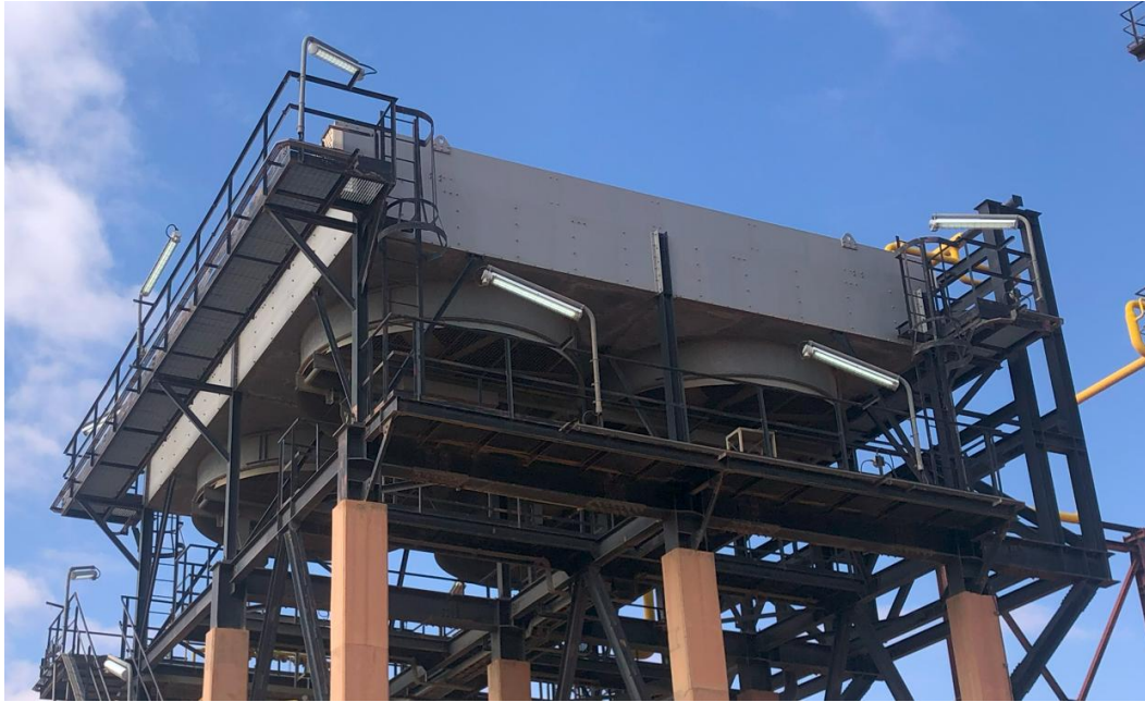
Figure II.7. Condensate Propane Cooling System.
