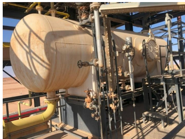
Figure II.3. Reflux Drum Used in Depropanizer Unit.
