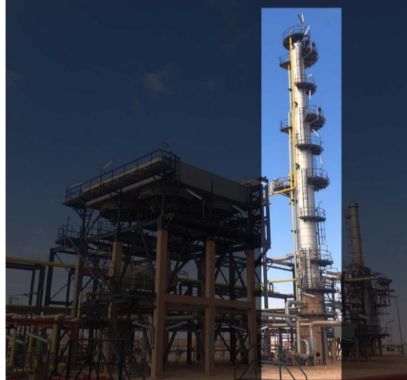
Figure II.2. Depropanizer Distillation in a Gas MPP3.
