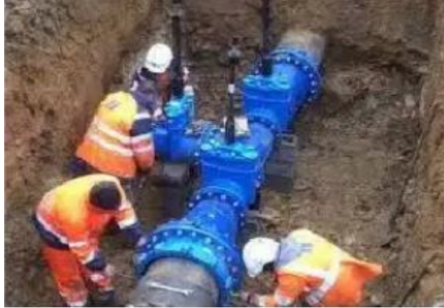
Figure II.40: Maintenance des infrastructures
