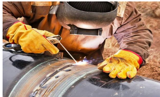
Figure I-9: Soudage MMA [29]
