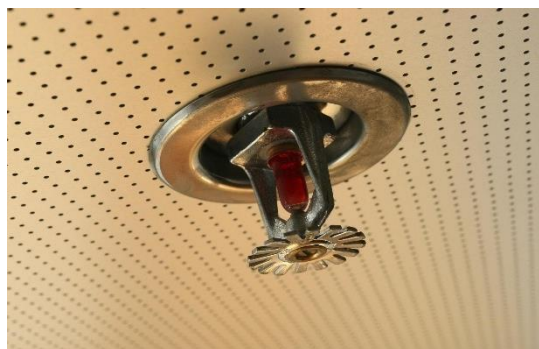
Figure 9 Sprinkler pendent[12]
