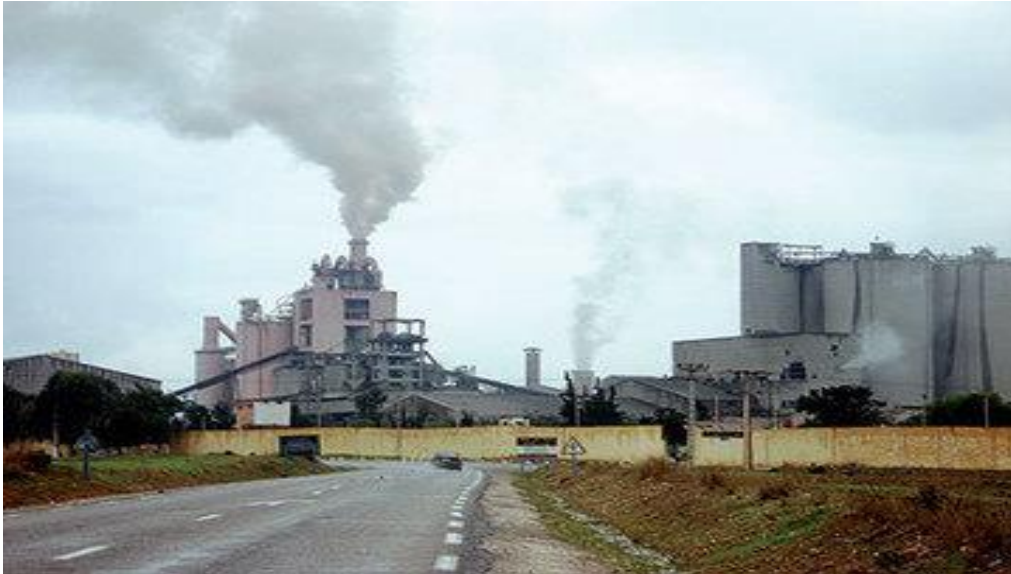
Figure 1.7: La cimenterie de Béni-Saf [8]
