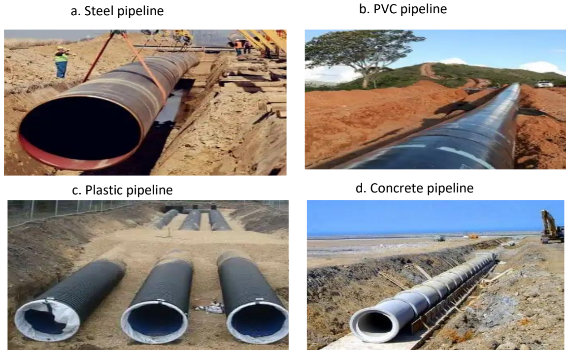
Figure 2- 4 Examples of some pipeline [28].
