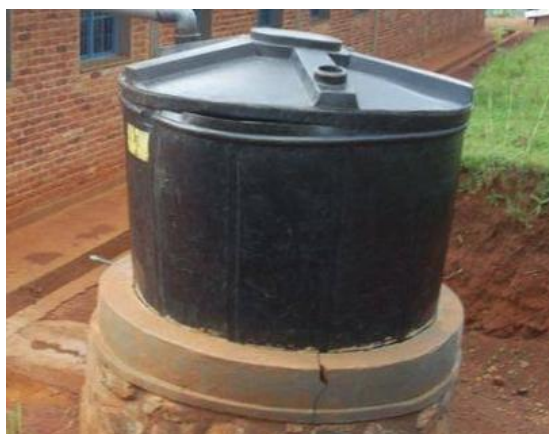
Figure 9: citerne de stockage
