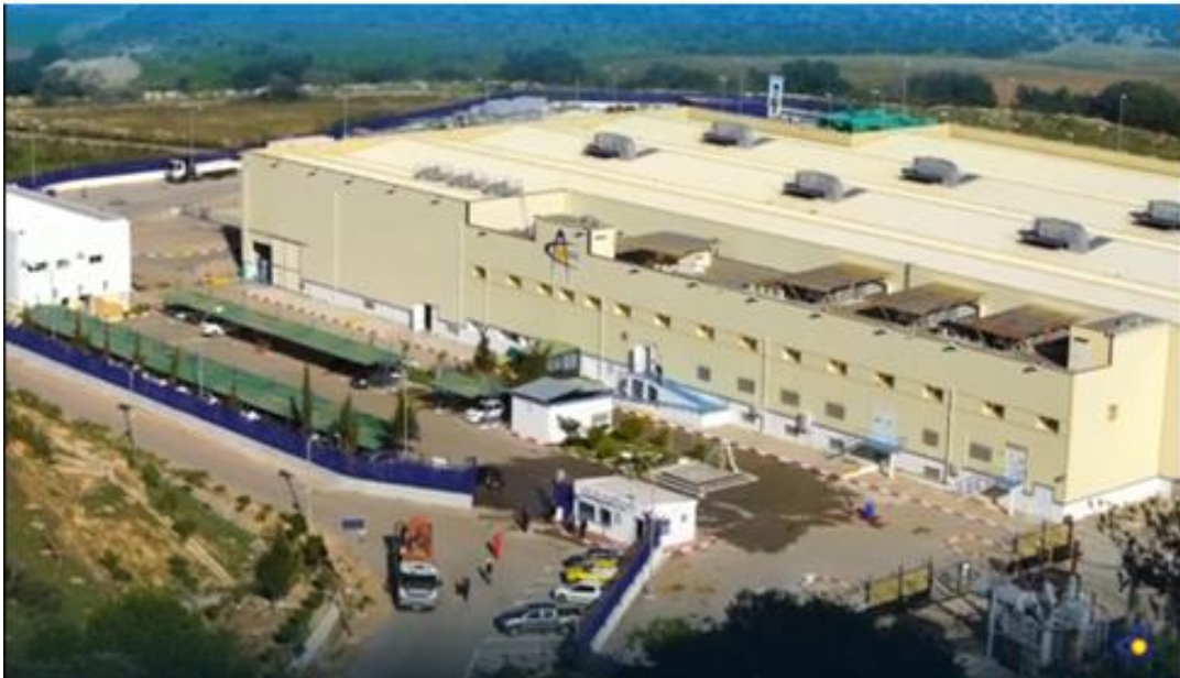
Figure II-1 : Station de Dessalement L'eau de Mer Beni Saf Water Company.
