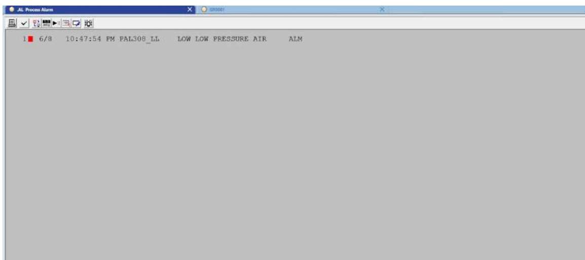
Figure IV.24. Process alarm view
