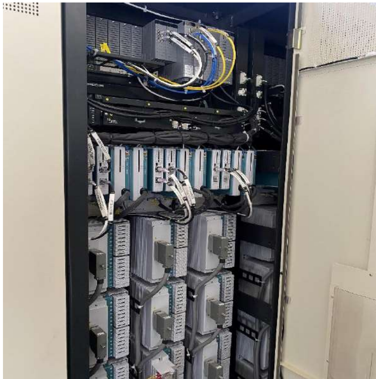
Figure III.1. Distributed Control System
