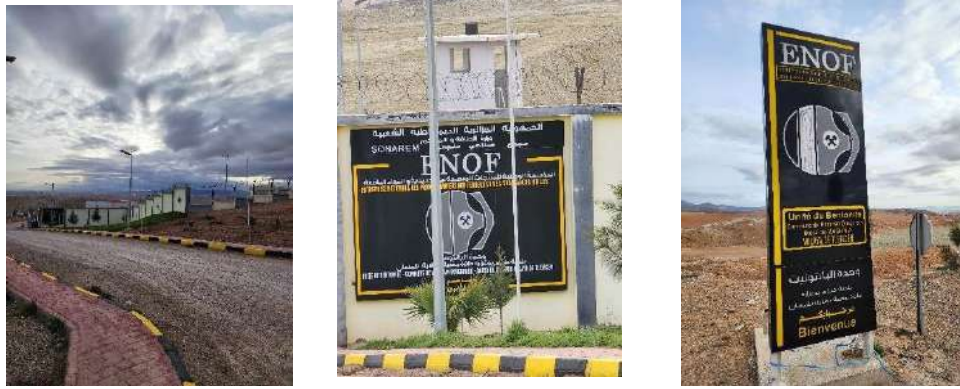
Figure 1.5 the Maghnia quarry (Hammam Boughrara)
