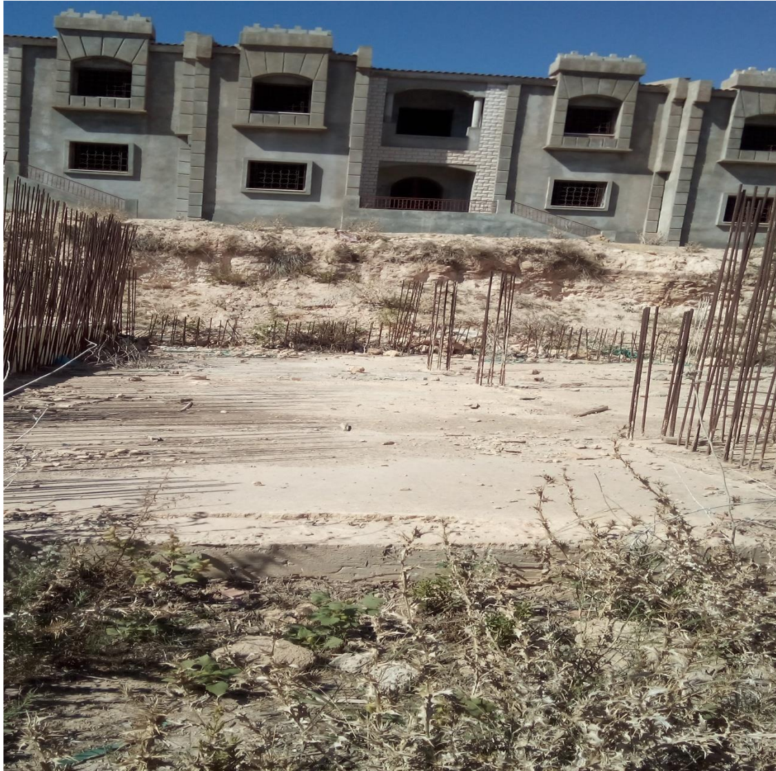
Figure IV.19 Photo Tuf de calcaire (83 villas AADL)-06/10/2019
