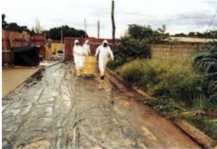
21. Much of the decontamination work had to be done in heavy rain.
