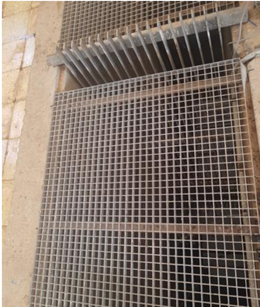
Figure III.5: Grille verticale mobile.
