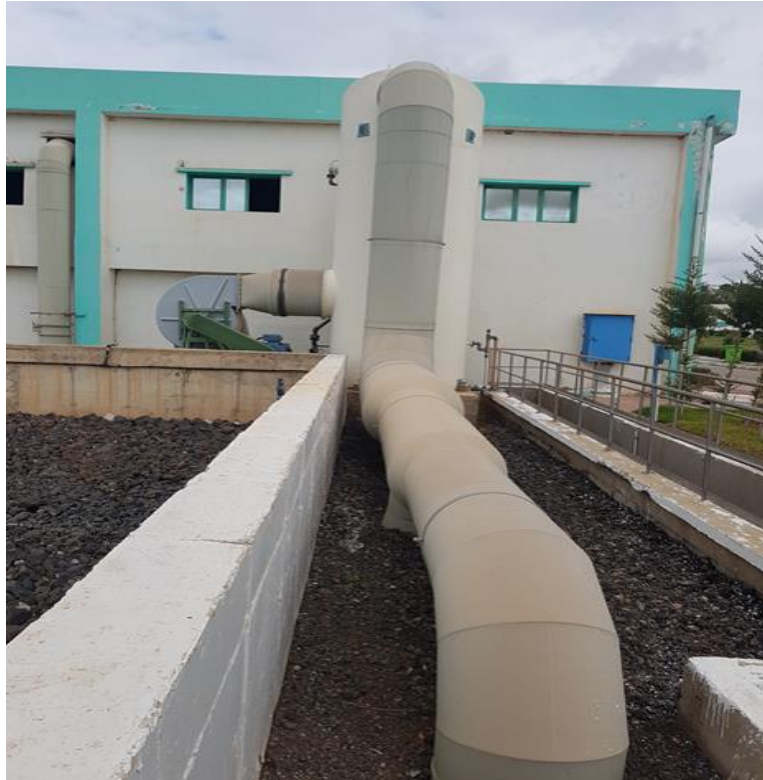
Figure III.25: Biofiltre ruisselant.
