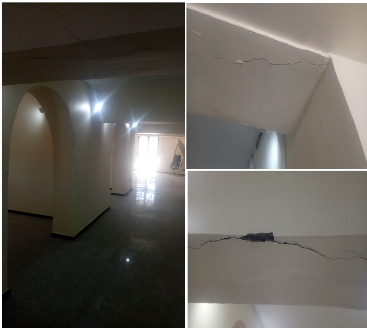
Figure I.60 : Fissures.
