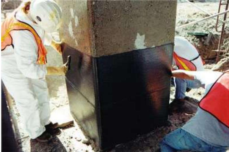
**Figure II.14:** Confinement de colonnes (Pantelides et al. 2002)
