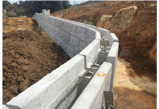
Figure II.19 Mur en cantilever (Youcef tani,2021).
