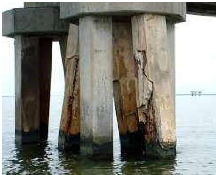
FIGURE 1. 7 DURABILITE DES PIEUX PREFABRIQUES EN BETON PRECONTRAIT EN
