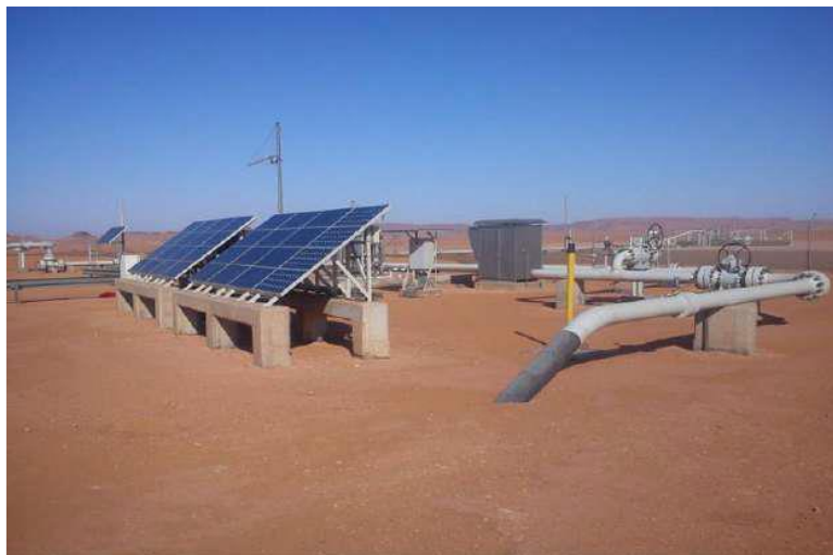
Figure I.1 : Installation photovoltaïque.
