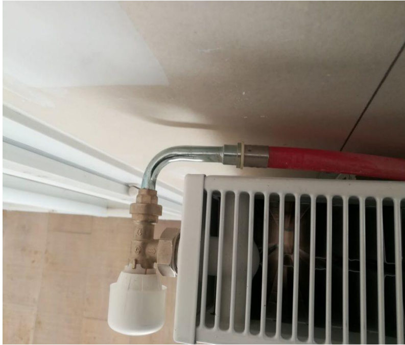
Figure 41: Installation en tube PER
