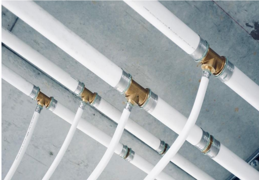
Figure 42: Installation en tube multicouche
