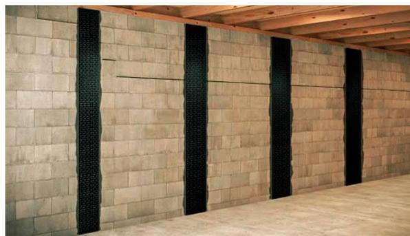
**Figure I.17:** Renforcement des murs. [10]
