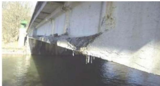
**Figure I.11:** Fissuration due au gel/dégel. [8]
