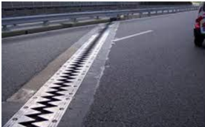
Figure 110: Joint de chaussée
