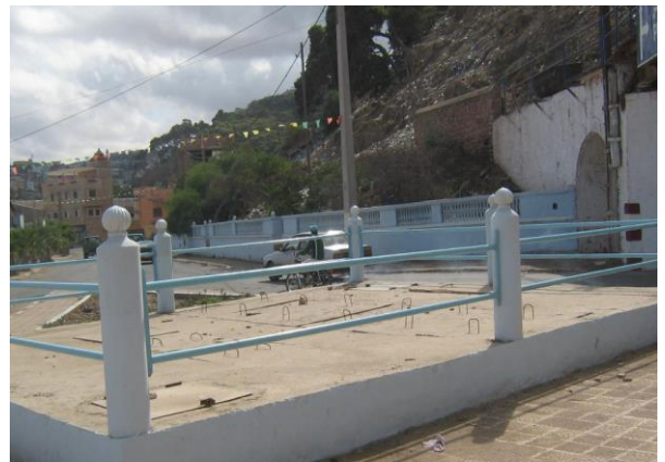
Figure N°V.3 :La station de relevage(DRE)
