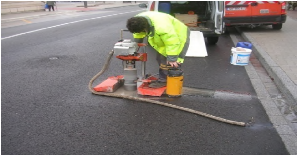
Figure III.7. : Carottage GRAVE Bitumineux 0/14
