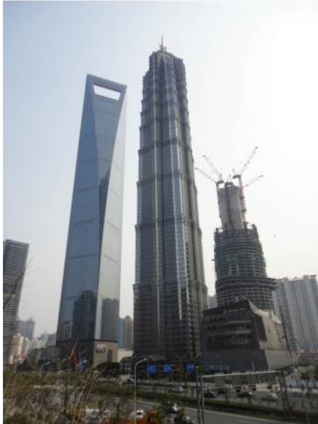
Figure III-4 : Shanghai Financial Center (la gauche), Jin Mao Building (centre), and Shanghai Tower en Chine (droite) En construction (photo by Kyoung Sun Moon).
