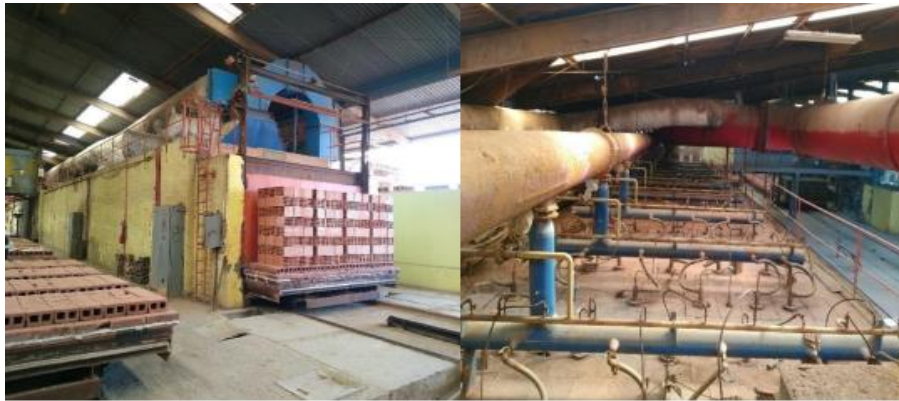
Figure 21 : Four a tunnel
