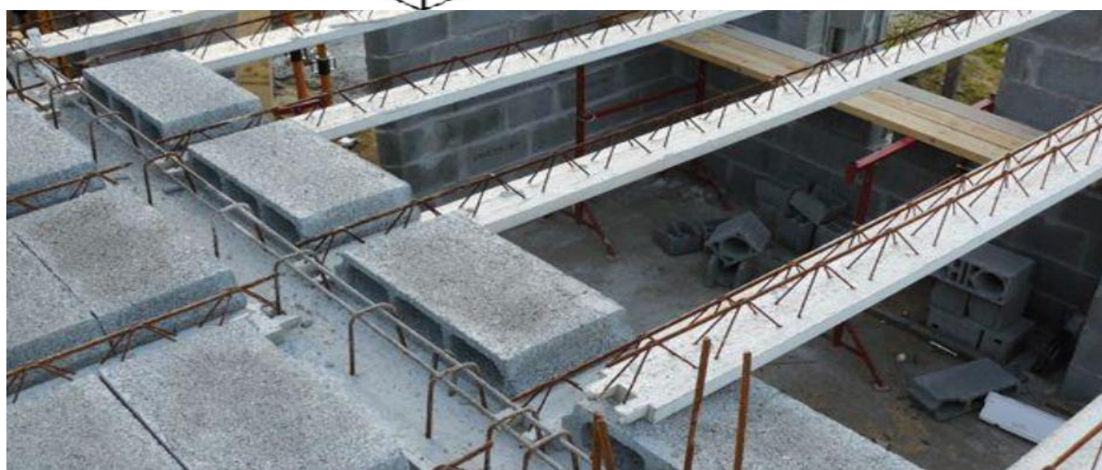
Figure I.16: dispositions des poutrelles
