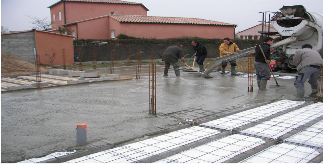
Figure I.20: Phase Coulage de la dalle.
