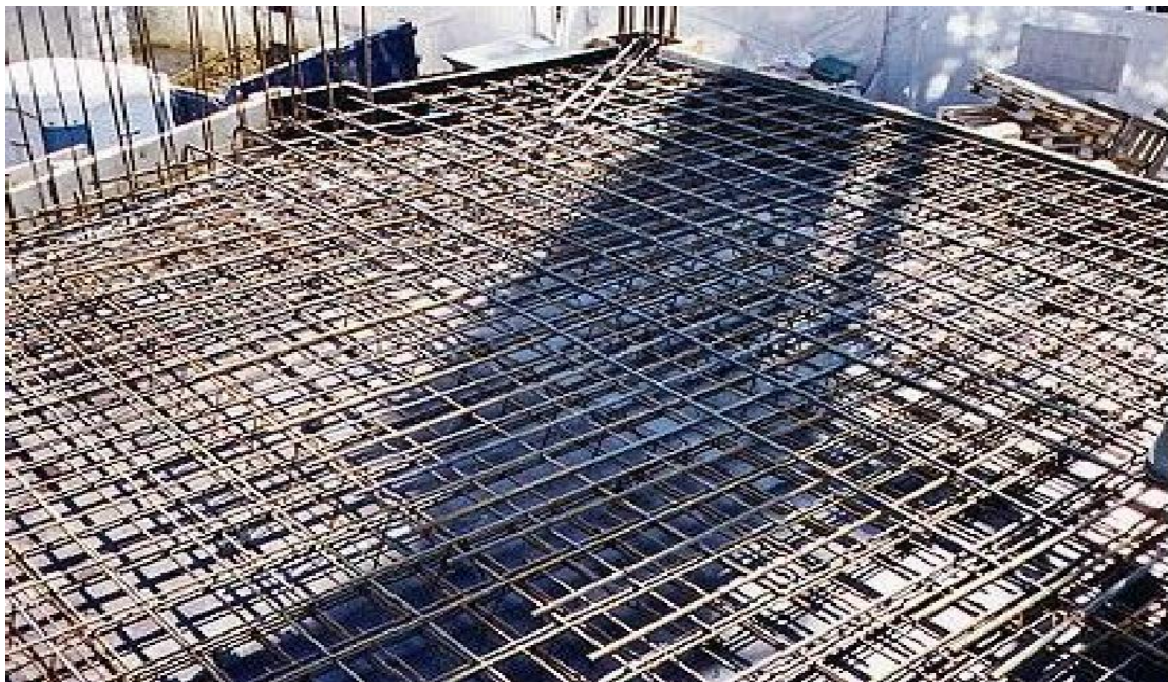
Figure I.22: Planchers en dalle pleine
