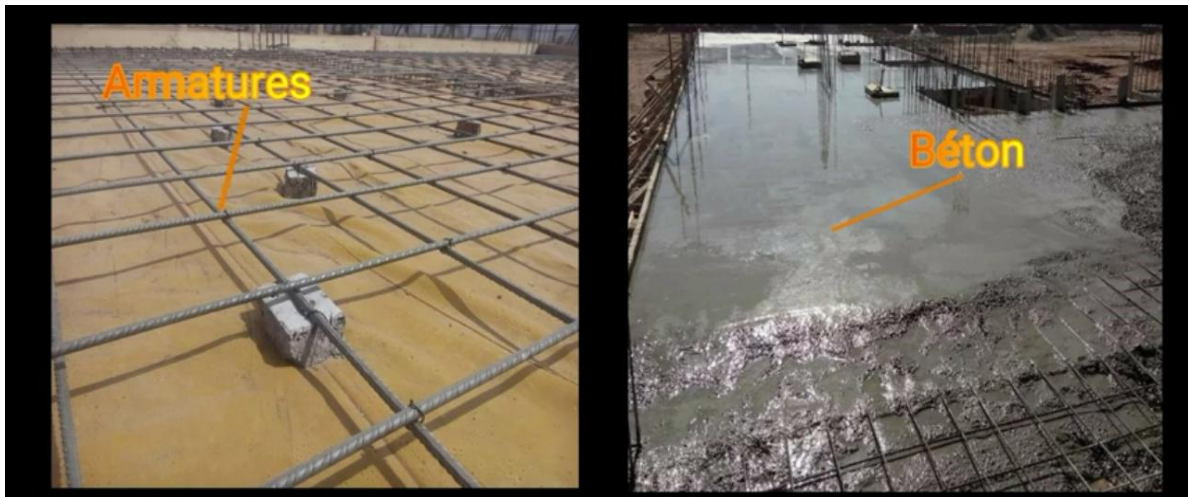
Figure I.25: les armatures dalle pleine
