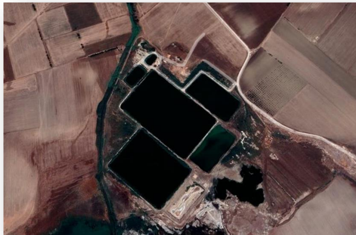
Figure 10: image satellite de station d'épuration d'Amria (ONA, 2021)
