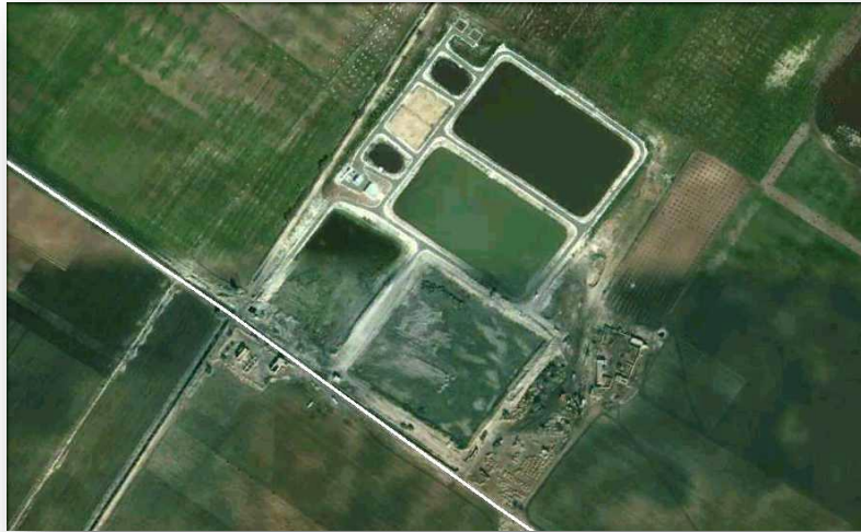
Figure 9: image satellite de la station d'épuration de Hassi Ghella (ONA, 2021)
