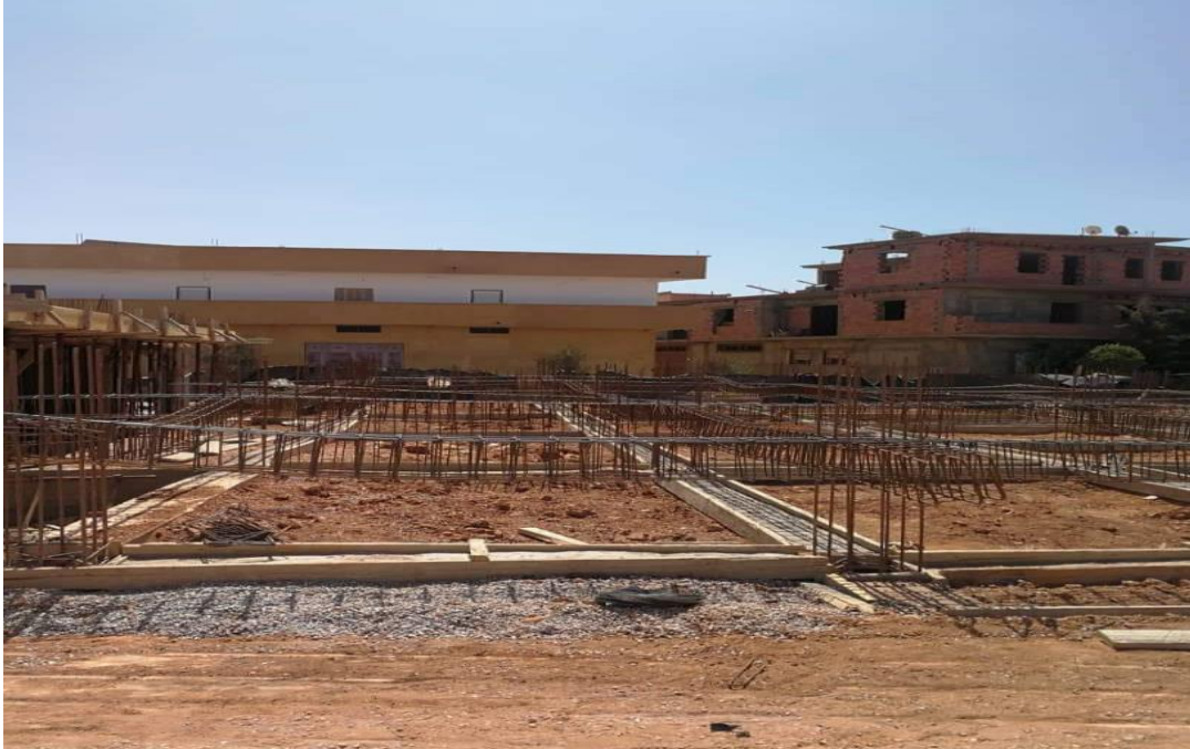
Figure 15: realisation des longrines
