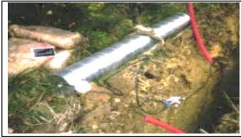
Figure II-23: ANODE PRÉBACKFILLÉE [29]
