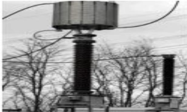
*Fig II-18 circuit bouchon*
